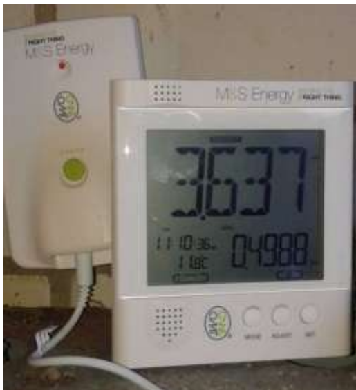
Figure 7: An OWL Electricity monitor (installed for trials in December 2014) will be used to collect energy usage data.
